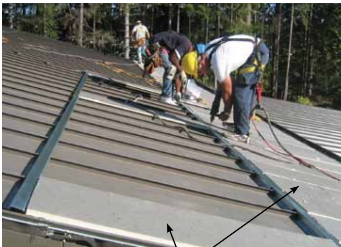
Roof Huggers being installed with rigid insulation.
