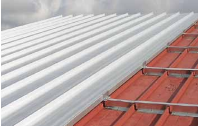
Vertical rib standing seam roof being installed over an old vertical rib standing seam roof.
