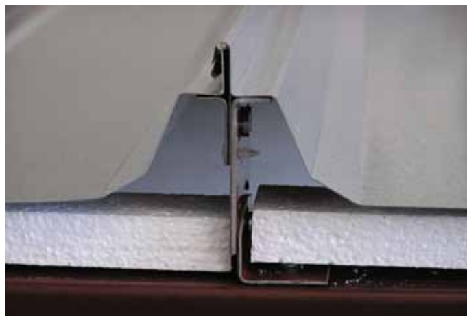
Typical standoff assembly for trapezoidal standing seam panel.
