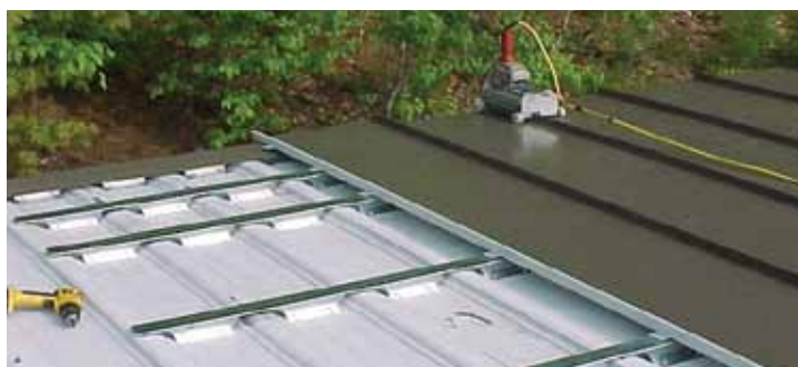
Vertical Rib Standing Seam over "R" Panel vented at the ridge
