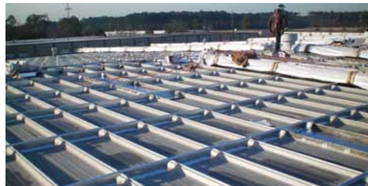
99,000 Square Foot Retrofit over existing Trapezoidal Standing Seam completed in 40 days
