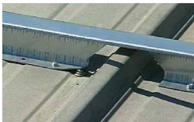
Existing fasteners usually do not have to be removed.
