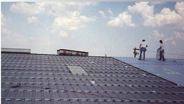
Roof Huggers make fast work of this 24,000 sq. ft. retro-fit project.
